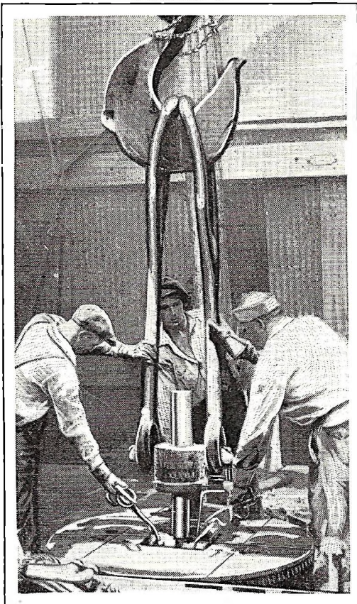
Lowering the drill pipe into the hole. The core barrel is fastened onto the lower end of the drill pipe and bites its 30-foot core far below the surface, whence it goes to laboratories where it is examined microscopically by geologists.
