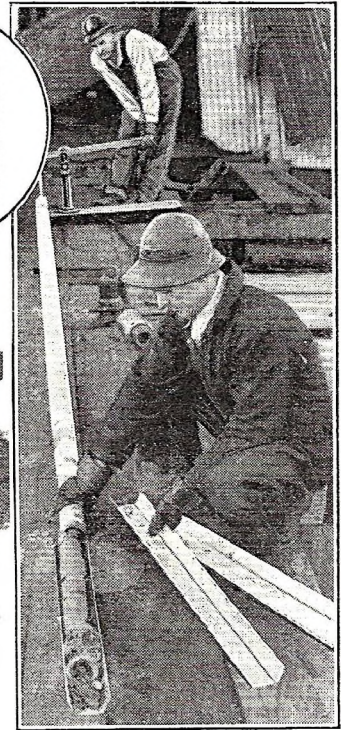
Geologist examining cores pulled from hole in earth 2 miles deep, to determine if the drill is near oil-bearing strata.
