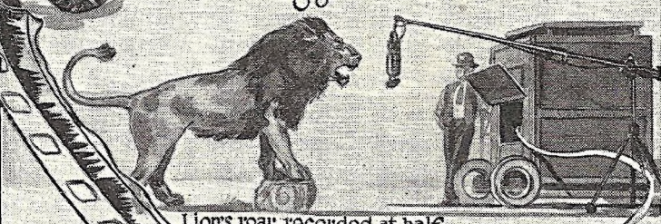
Lion's roar: recorded at half speed and printed in reverse on sound track gives terrifying cry of prehistoric beast
